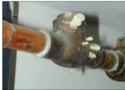
Growths on brass fitting associated with microbiologically influenced corrosion.
